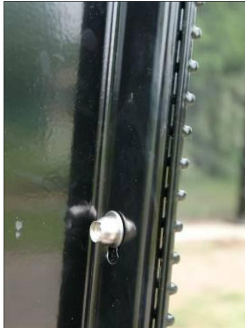
Finally secure the upper 4 bolts incl. cap & cover plate on middle and end post
