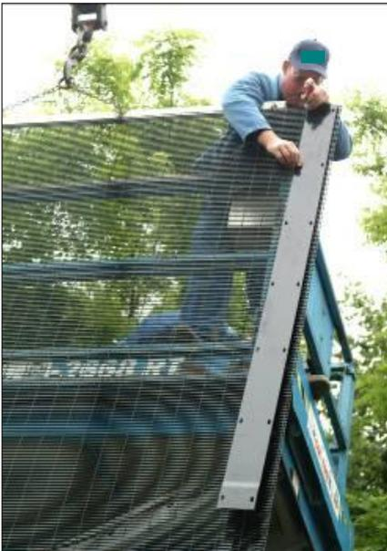
Fix temporarily by means of bolts while holding the panel in position with the crane
