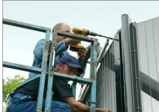
Finally secure the 4 upper bolts at left and right side whilst holding the panel in position with the crane
