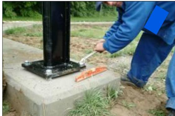
Leveling by means of nut & contra-nut
